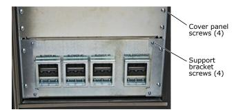
**6.** Remove 25IP Torx+ screws (4) that attach the cover panels above the front of the PDU and remove the panels.
