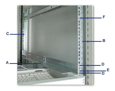
Figure 29: Installing the right support rail
